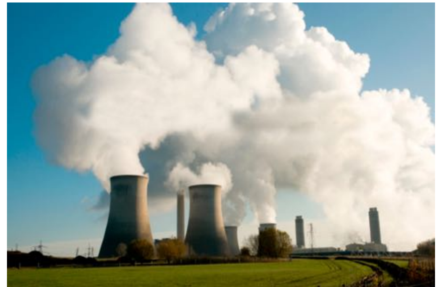
WET COOLING TOWERS
